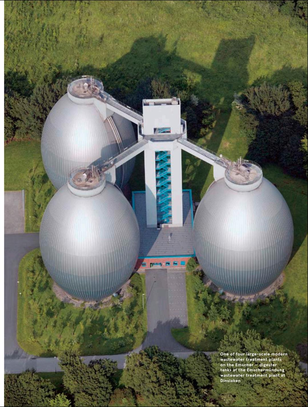
One of four large-scale modern wastewater treatment plants on the Emscher – digester tanks at the Emschermündung wastewater treatment plant at Dinslaken
